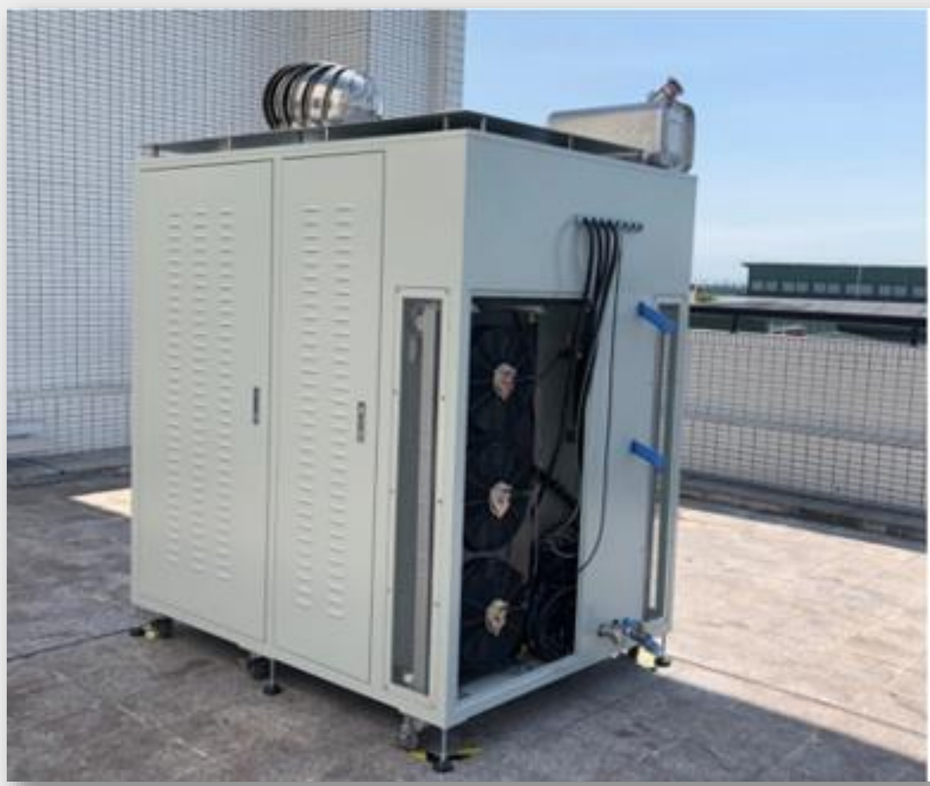
50 kW fuel cell system using industry H 2 bi-products
