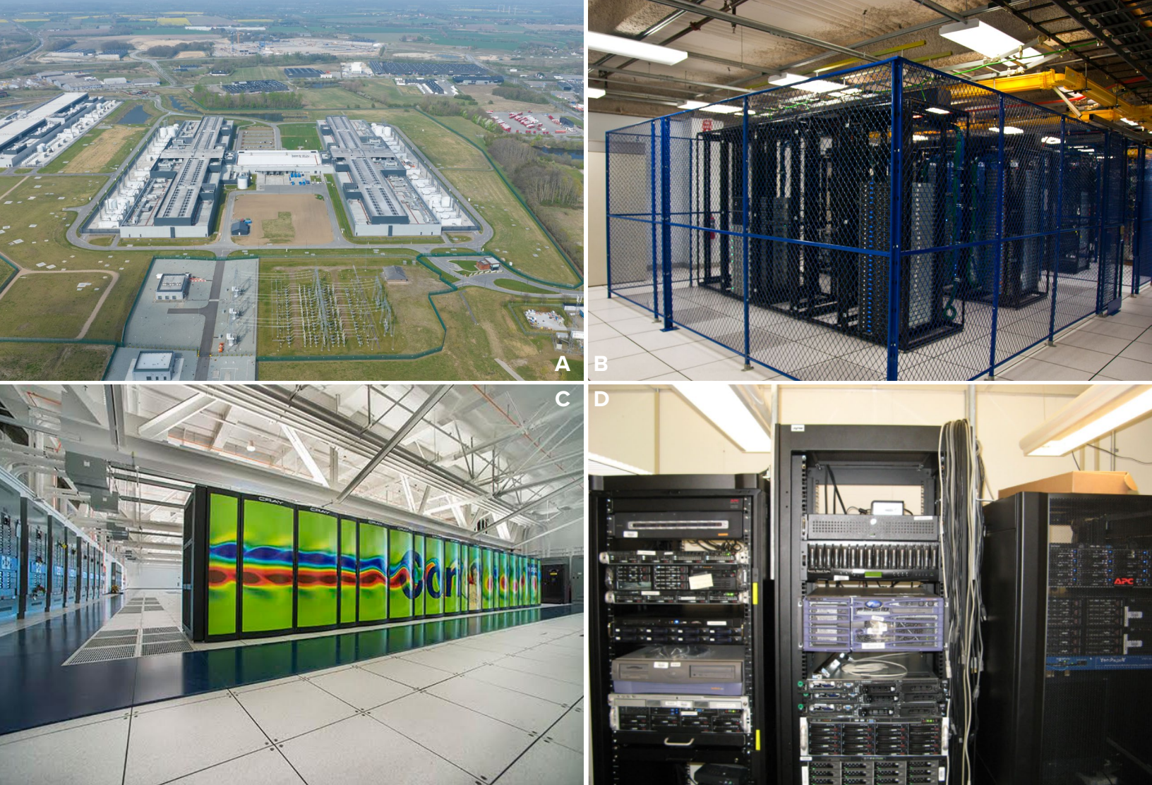
Figure 1-1. The many shapes and sizes of data centers: (a) Meta's hyperscale data center campus in Odense, Denmark, which contains more than 200,000 m 2 of floor area 10 ; (b) an example of a tenant-leased space in a co-location data center with secured access 11 ; (c) a high-performance computing (HPC) data center occupying around 13,000 m 2 12,13 ; and (d) a small data center room in an office building, occupying less than 100 m 2 14 .
