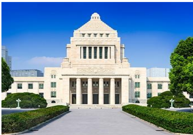
National Diet Building -- Tokyo, Japan
