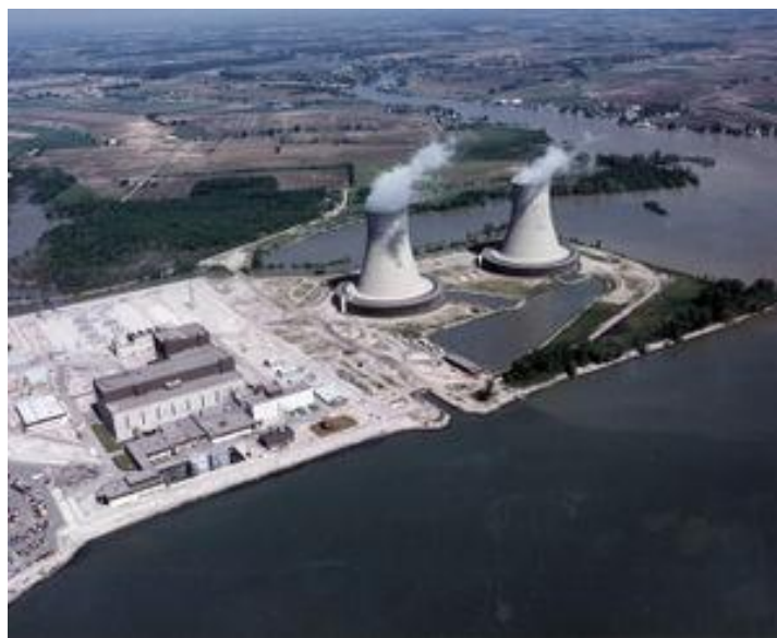
Figure 10-1. Boiling water reactors at the Enrico Fermi Nuclear Plant in Newport, Michigan, USA. 9
