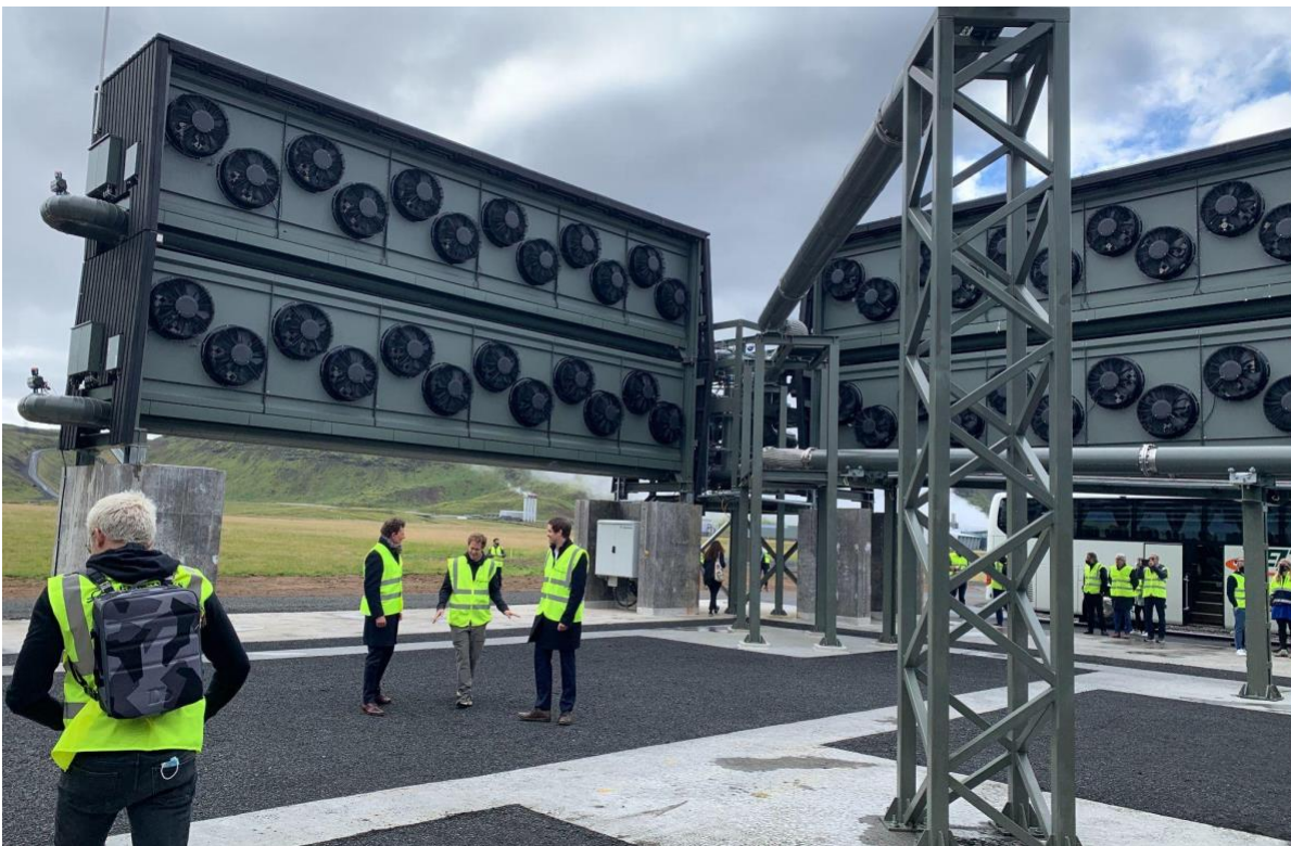
Innovative materials are important for enabling carbon capture and removal systems, such as this direct air capture (DAC) plant in Iceland (photo credit: Julio Friedmann).
